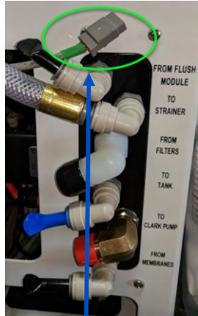
Z-ION Connector (with green band). Left unused if your system was not ordered with the optional Z-ION.
