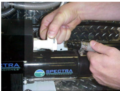
Connecting brine discharge service hose
